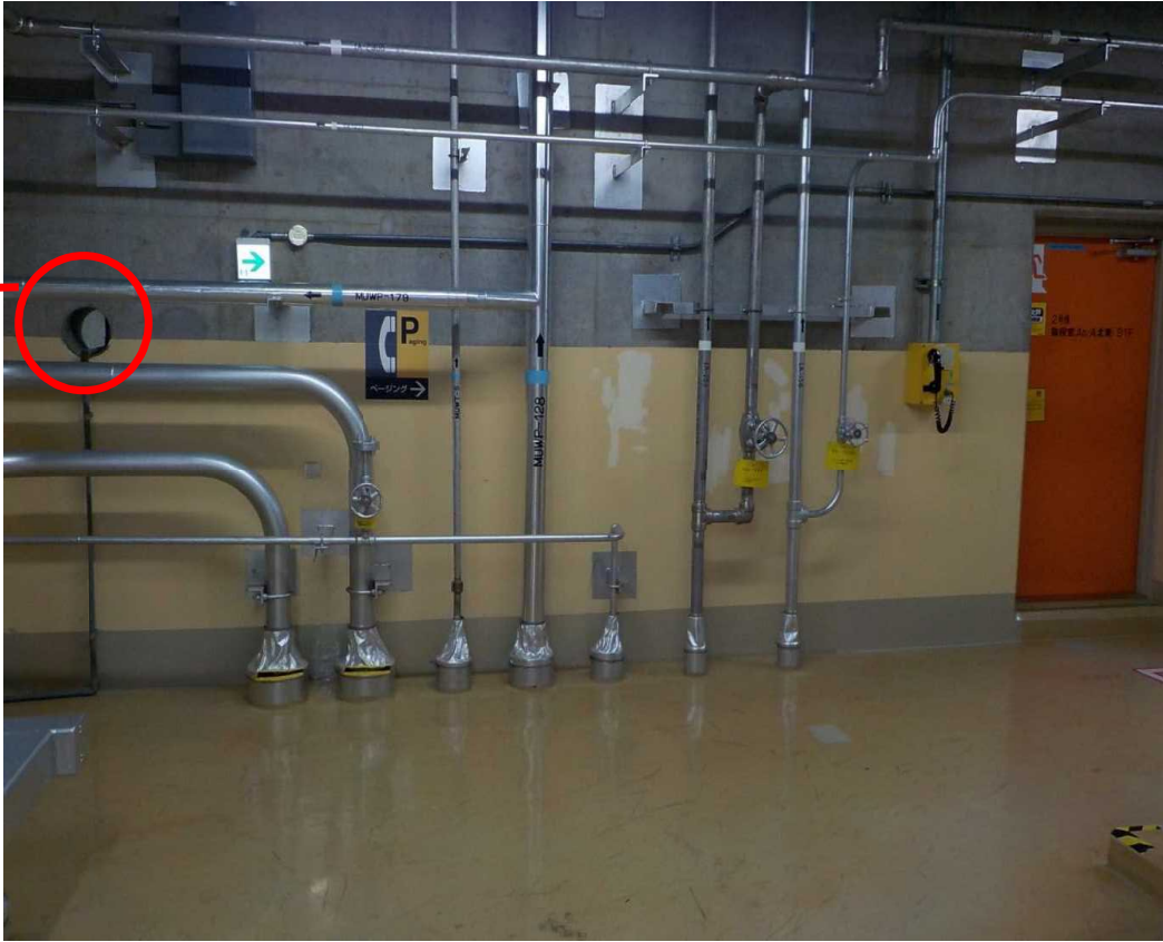
地下1階北東廊下側
