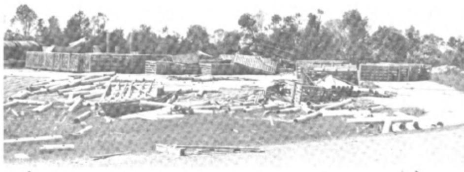
パイプを収納した木箱（一部 2 段重ね）は浮上せずに転倒し、パイプが周囲 7m~9m に散乱 (Pieces of pipe were scattered over the area, but none travelled more than 25-30ft. The pipe joints are 8in. dia. x 8ft. long.)
